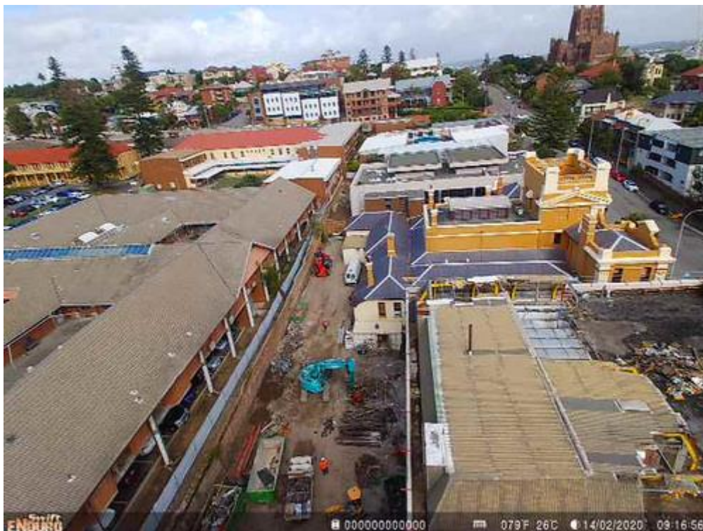
Photo 01: Initial time-lapse photo of the site taken on 14/02/2020
