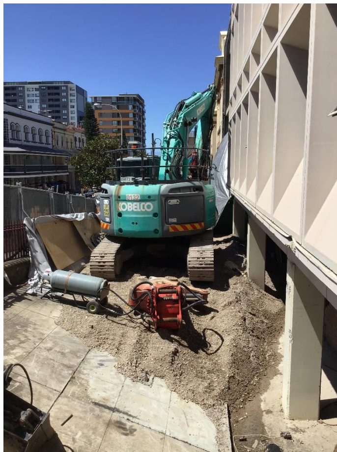
Photo 19: View from front of Supreme Court Building facing East. Note road base/aggregate for plant platform due to existing slope conditions.
