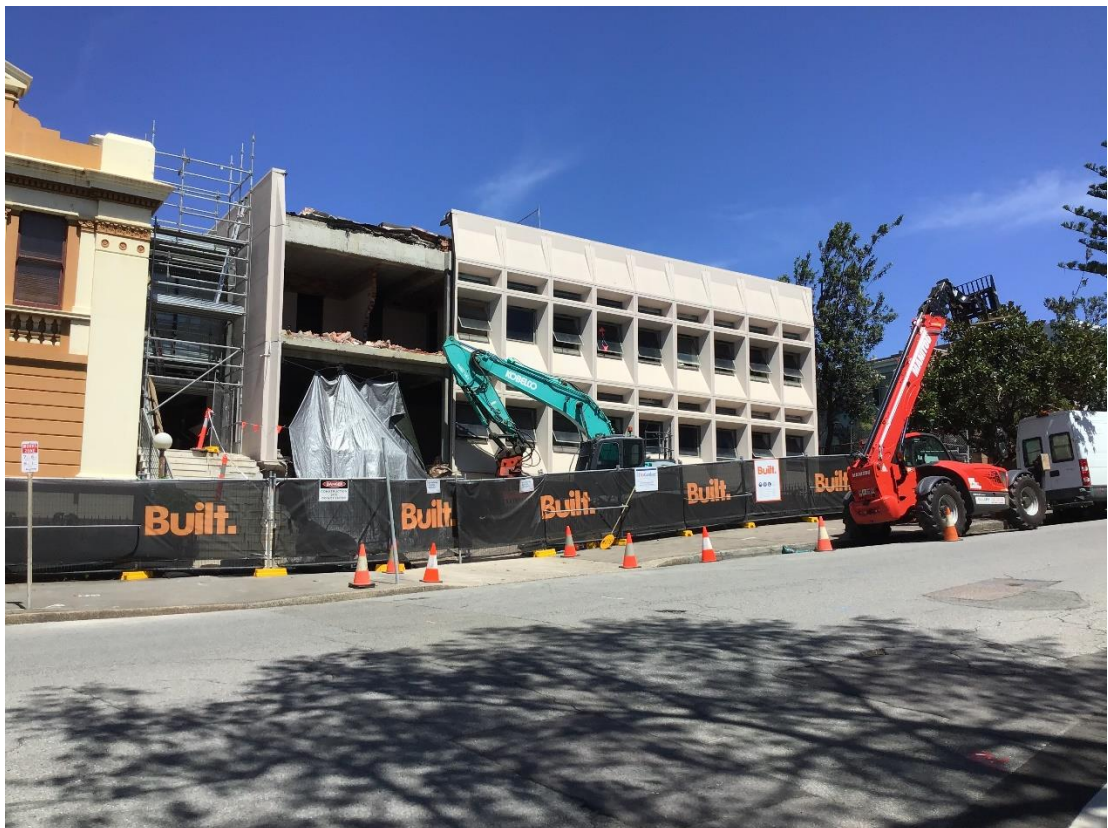
Photo 06: View of site from the opposite corner of Church & Bolton Streets. Note opening formed to allow for removal of soft strip materials into a bin below.
