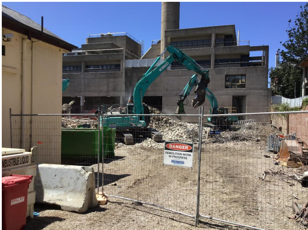
Photo 11: View from rear of Courthouse facing East showing heavy demolition plant. Note the exclusion zone in place.
