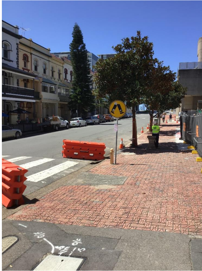
Photo 07: View from site access door facing East showing Work Zone, pedestrian protection barriers and Traffic Control personnel.
