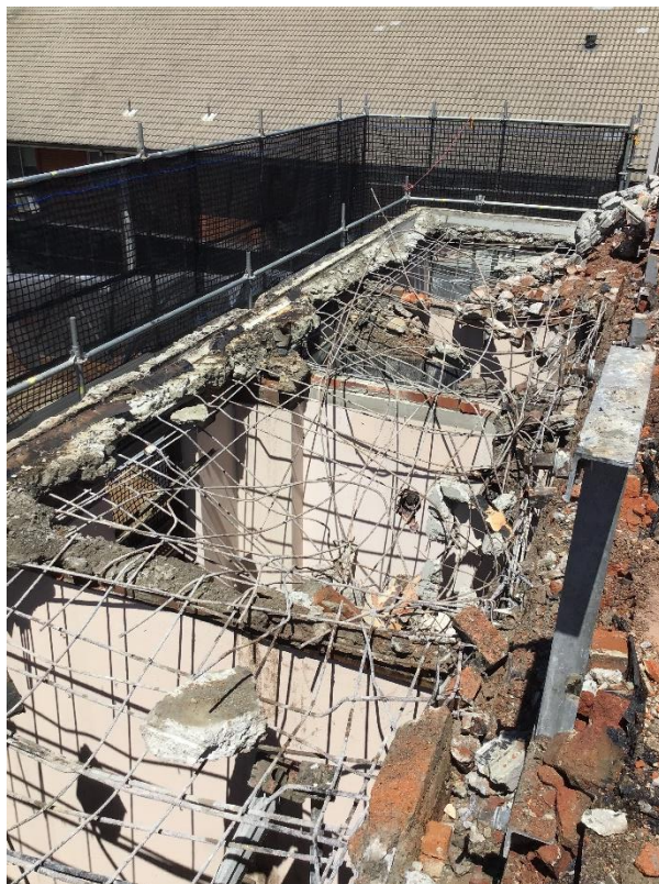
Photo 17: View from the rooftop of the Supreme Court Building showing the demolition of connection between Heritage & Supreme Court Buildings. Note scaffold to protect heritage structure.
