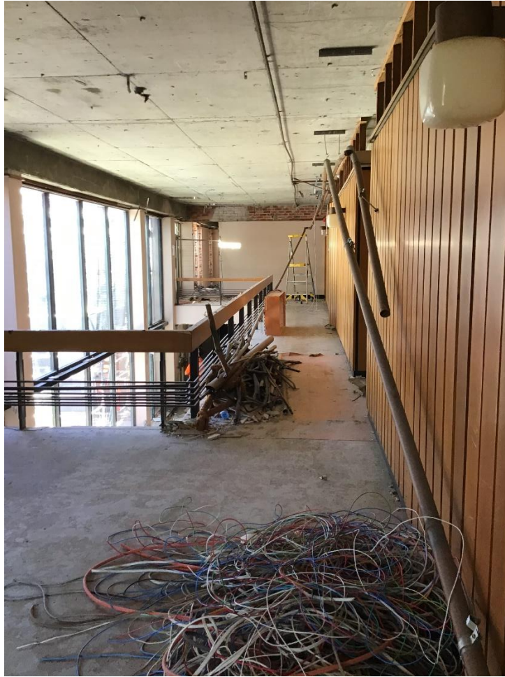
Photo 20: Internal view from Level 3 showing soft strip demolition works. Note Levels 1 and 2 were inaccessible due to intensive demolition works
