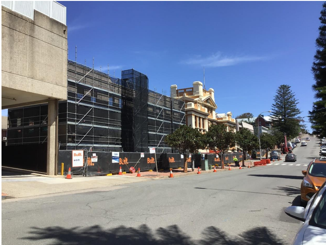
Photo 03: View of site from Church Street facing South West showing Demolition Scaffold & Work Zone
