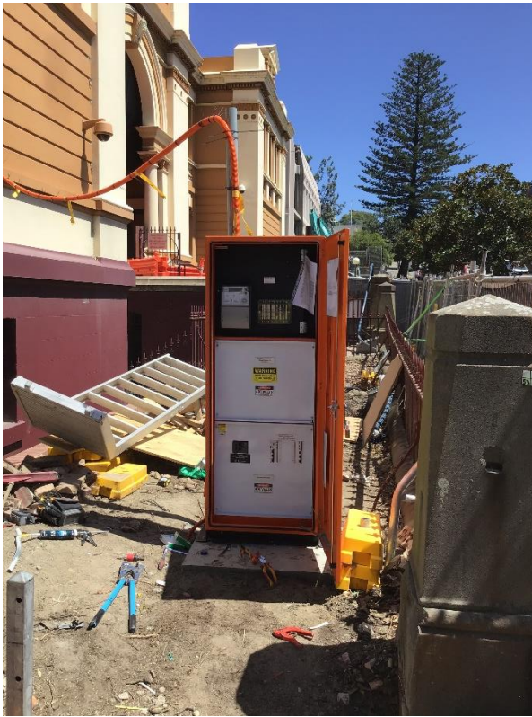
Photo 09 & 10: New temporary Electrical Distribution Board installed and existing removed. Inspected and approved by Ausgrid on 28/02/2020
