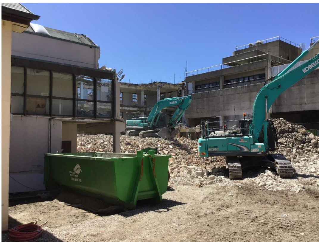
Photo 12: View from rear of the site facing North showing heavy demolition to Administration Building
