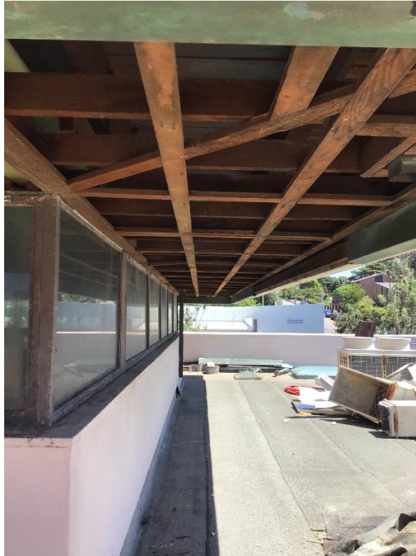
Photo 16: View from the rooftop of the Supreme Court Building showing asbestos removal from eaves.
