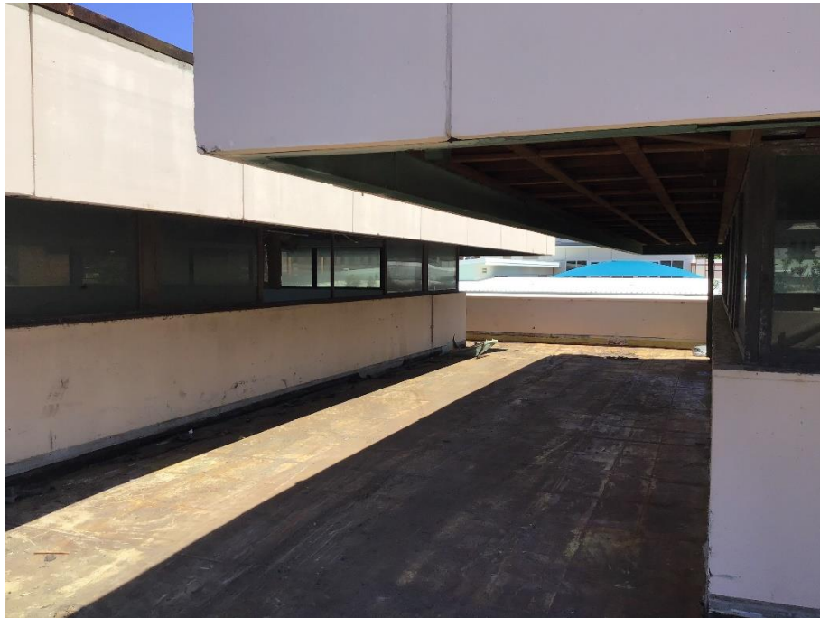
Photo 18: Supreme Court Building rooftop showing roof coverings and asbestos removed.
