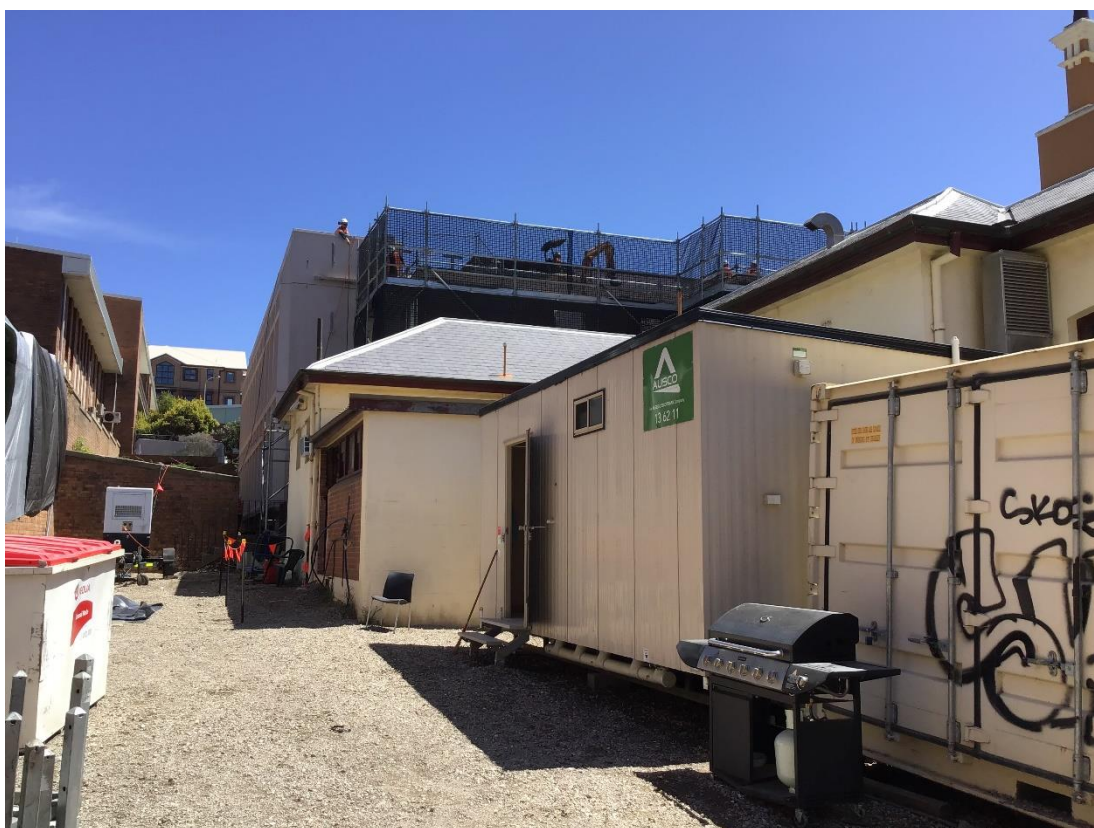
Photo 14: View from rear of Courthouse facing West showing Demolition scaffold to Supreme Court Building
